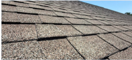
5. Shingle field on an accessible plane. Dry surface with moderate localized granule loss.
