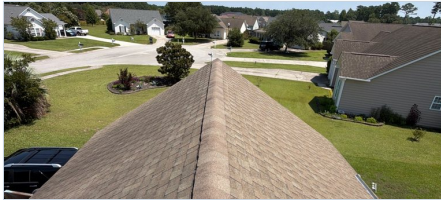
4. Main hip ridge running the length of the roof.
