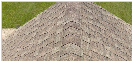
11. Rear hip ridge and roof planes above the back of the home.
