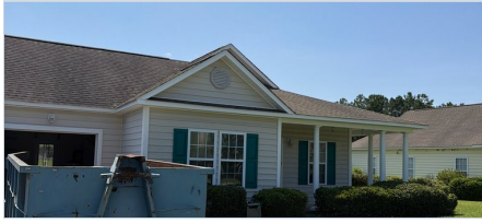
1. Front elevation. Architectural asphalt shingle across multiple planes.
