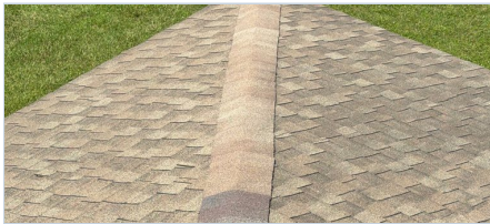
7. Ridge cap wear and color variation along the hip.
